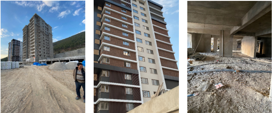
Image 6. In Kahramanmaraş, three 15-story blocks with large shear walls and a shear wall-frame structural system did not experience any structural or non-structural damage following the February 6, 2023, Kahramanmaraş-Centered Earthquakes
