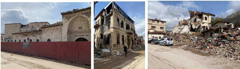
Image 3. Damage to Some Masonry Structures and Collapsed Masonry Buildings in Hatay Province (left image: Habib-i Neccar Mosque)
