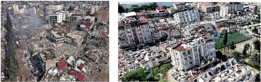
Image 1. Views of Collapsed and Completely Destroyed Buildings (left: Kahramanmaraş Province https://www.nytimes.com ; right: Hatay Province https://www.eeri.org )
