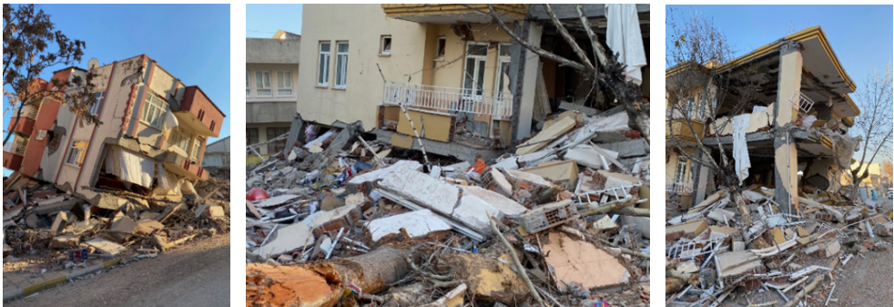
Image 2. Buildings Completely Collapsed Due to Soft-Story Irregularities on the Ground Floor
